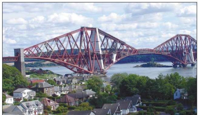
Firth of Forth Railway Bridge
